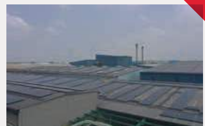
Rooftop Solar, MIL Rohad
