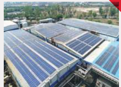
Rooftop Solar, MIL Hapur
