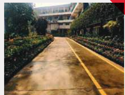
Merino Factory, Administrative Section, Hapur
